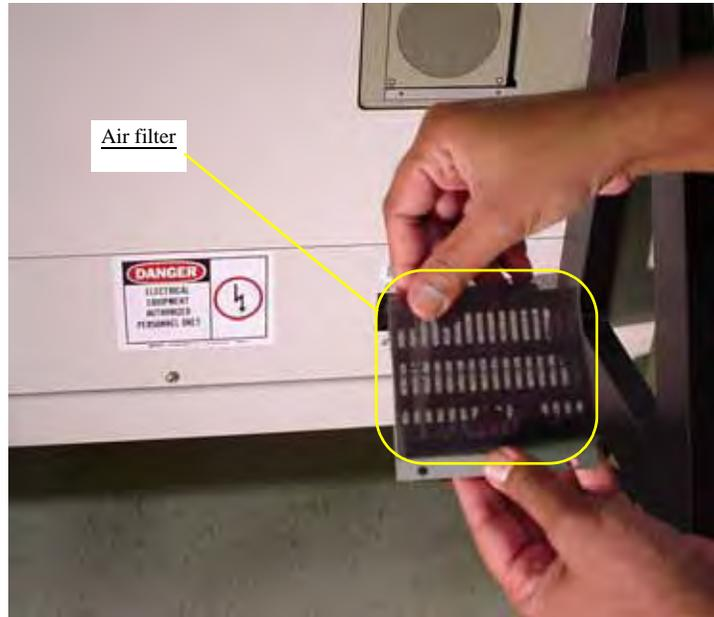
Figure 5-22—Replace air filter
